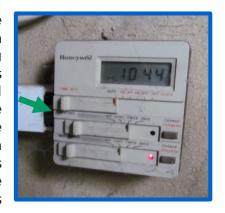
2) <u>Set heating time to match usage</u> - There were no bookings in the building for the morning of the assessment visit however the heating was on, presumably on the 'twice a day' setting. Matching heating times to building usage, reducing the heating to a low setting such as 10 to 12°C between bookings, will reduce energy use.
